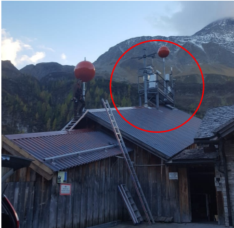
Abb.1: TAWES Station in Kolm Saigurn auf der Talstation der Sonnblick Seilbahn Fig.1: TAWES station in Kolm Saigurn at the roof of the valley station of the Sonnblick cable car. Quelle/Source: G.Holleis/SV
