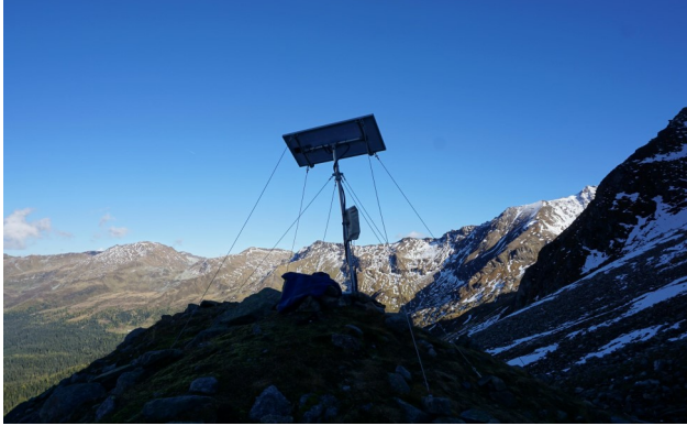
SeisRockHT MOR-Station am Fusse der Sonnblick Nordwand. SeisRockHT MOR- station at the foot of the Sonnblick north face. Quelle/Source: GEOSPHERE AUSTRIA/Binder
