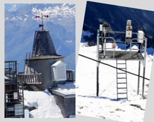
Abb.2: TAWES am Sonnblick Observatorium Fig.2: TAWES at the Sonnblick Observatory Quelle/Source: GEOSPHERE
