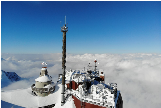
Abb.1: Sonnblick Observatorium am Hohen Sonnblick Fig.1: Sonnblick Observatory at Mt. Hoher Sonnblick Quelle/Source: L.Rasser@GeoSphere-SBO
