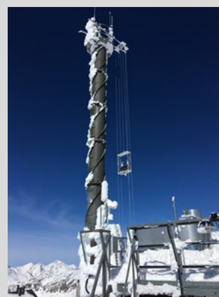
Elevator with the Holographic Imager at the Sonnblick Observatory Quelle/Source: A. Beck
