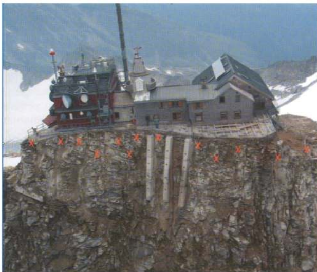
Illus.1: Placing sensors on the north flank of the Sonnblick summit
