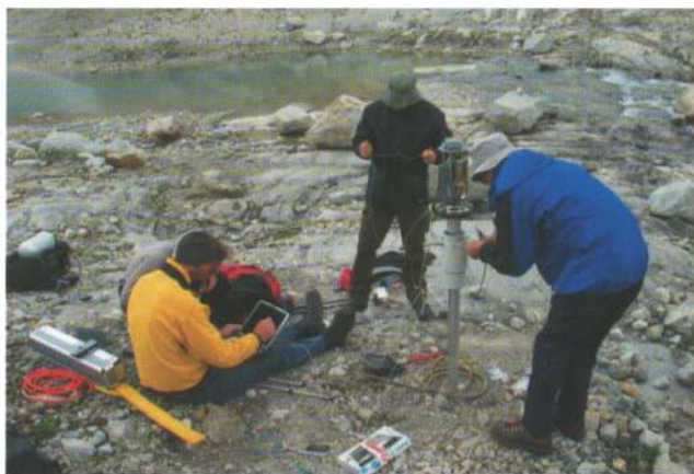
Illus.1: Installing a runoff gauge
