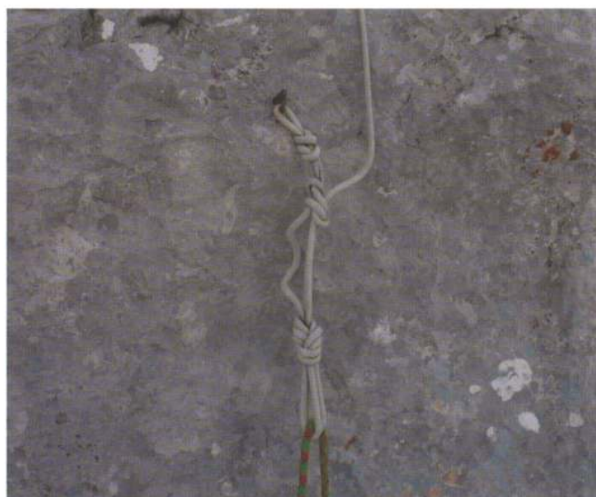
A polyamid rope rapelling stand, about 20 years old.
