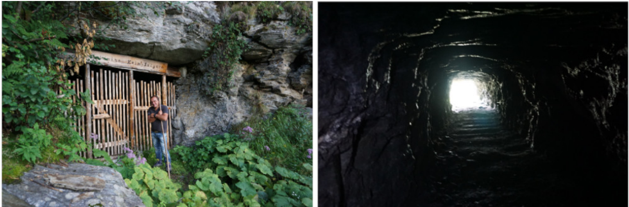
Figure 3.24: The tunnel portal and the \sim 50 m long tunnel. The GPS antenna is mounted on top of the tunnel portal.
