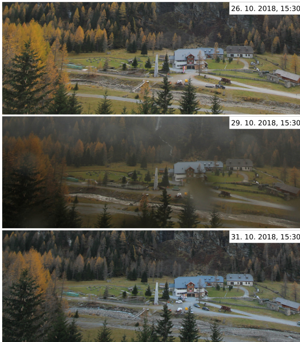
Figure 6.20: Photo time series of a mud flow coming down the river bed of the Hüttwinklache. The top photo shows the river bed before the heavy precipitation event, the middle the rising discharge, and the bottom photo documents the mud flow deposit and river bank erosion after the extreme weather event in October 2018. Based on the time lapse photos the mud flow happened in the night 29.-30.10., which corresponds well with the second precipitation maximum of this weather event (compare Figure 6.18). Source: foto-webcam.eu
