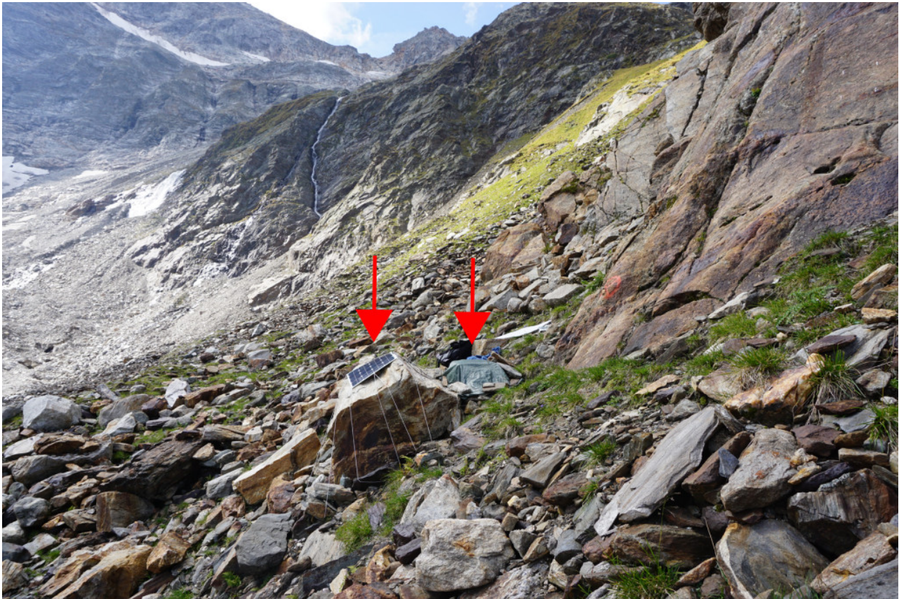
Figure 3.41: The temporary PIL station in late summer 2018. The left arrow points at the semi-flexible solar panel (50 W) fixed with cord on the rock. The right arrow points at the with a green tarp covered battery and data recorder boxes.
