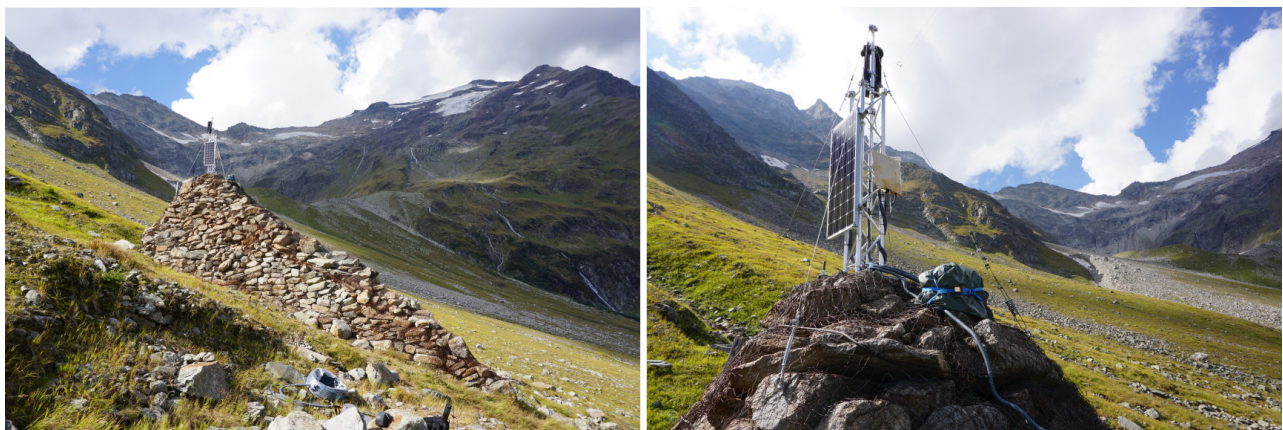
Figure 3.31: The avalanche wall above the old cable car pillar 'Mittelstütze'. The new MIT station was installed on top of the avalanche wall. The original battery box (wrapped in a green tarp) was situated in the lower right corner. The new battery enclosure was mounted right below the original battery box.
