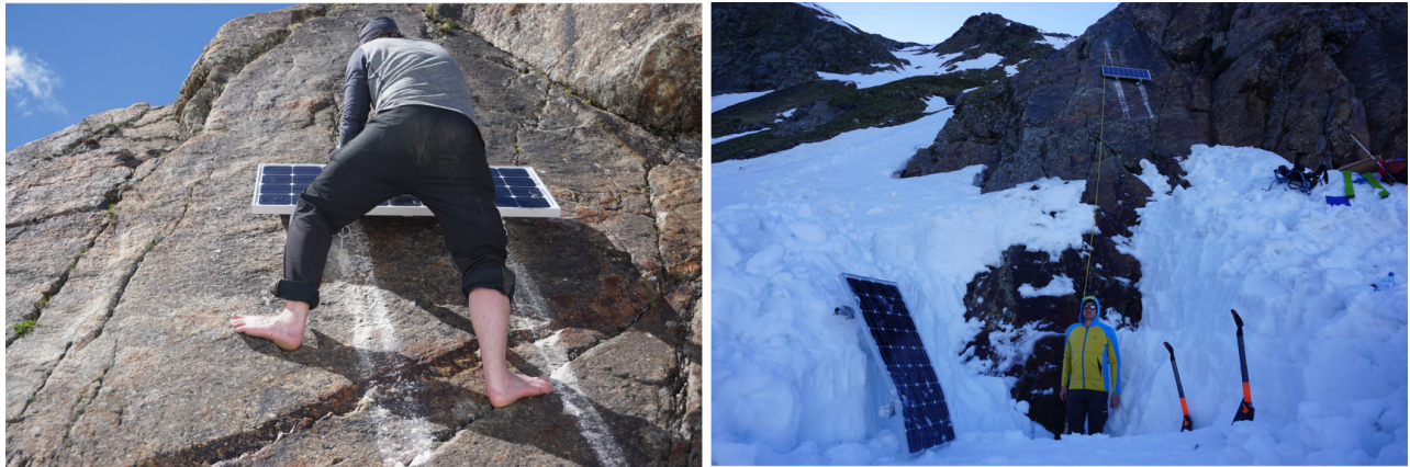
Figure 3.38: In May 2017 a new solar panel was mounted at about 10 m above ground. In the foreground of the right image the recovered wrecked solar panel can be seen. The background shows the new solar panel mounted on the upper rockwall. Furthermore, the image gives an impression of the snow masses accumulated over winter which had to be removed to actually recover the old solar panel.
